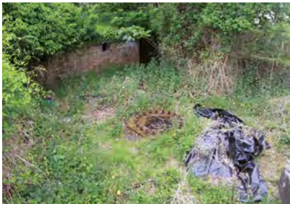
Figure 38. Unusual gunhouse at Hollesley that housed one of a pair of 6-inch guns intended to give artillery support to Harwich Haven. The holdfast for the gun can be seen in the middle.
