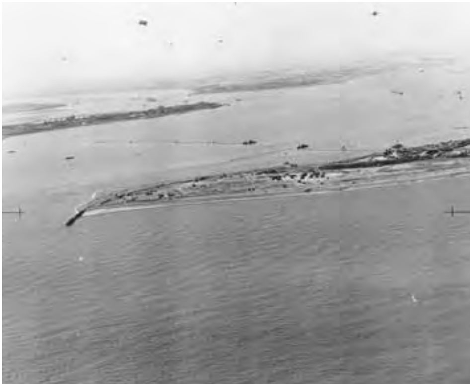
Figure 22. The mouth of the Orwell in 1941, showing the boom across the river and barrage balloons tethered to ships. In the foreground, Landguard Point is covered with anti-invasion defences. (English Heritage, RAF Photography)
