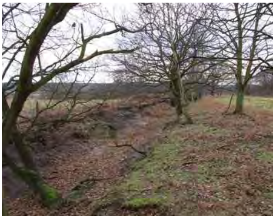
Figure 22. Anti-tank ditch at Walberswick showing the distinctive 'V' profile.
