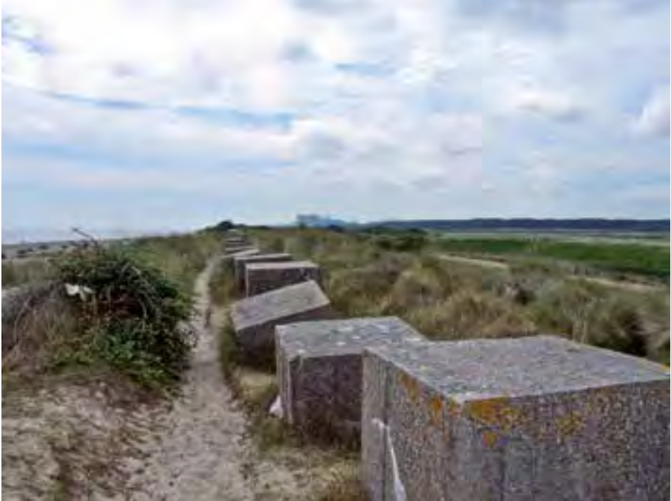
Figure 60. Anti-tank cubes, Minsmere Levels. Here the long run of blocks formed a continuous obstacle.
