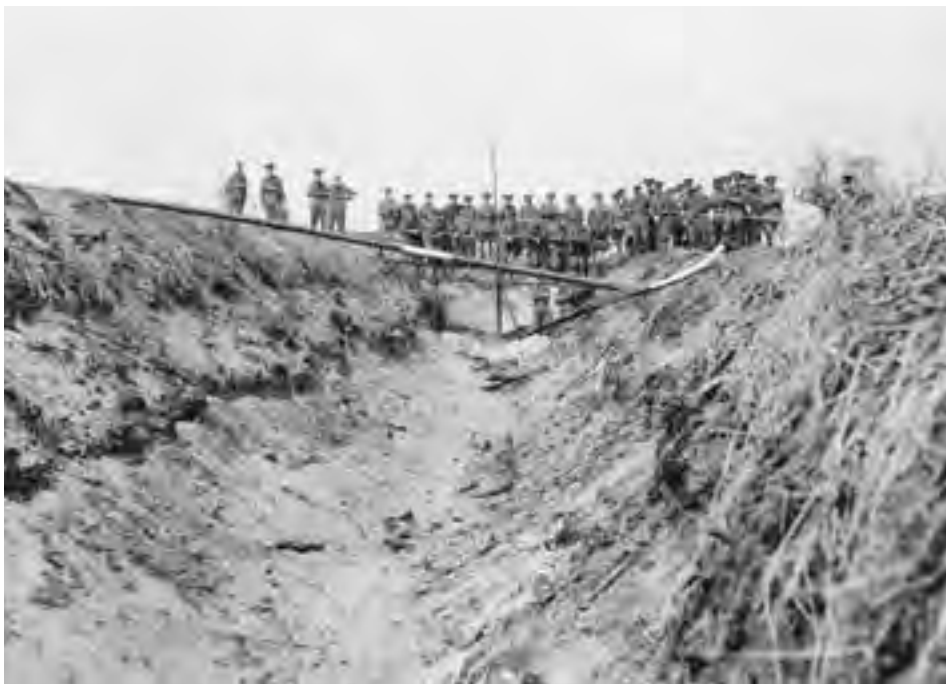
Figure 42. Senior officers watching a demonstration of the 'Snake', an explosive device used for clearing a passage through minefields and barbed wire. (IWM H 29057)
