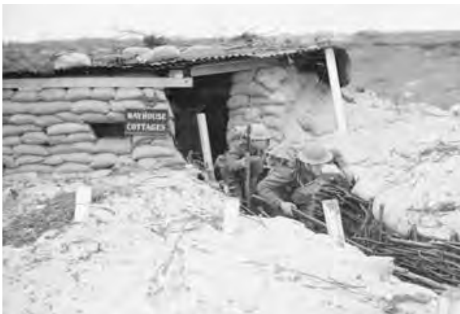
Figure 35. This image shows an improvised dugout made from timber, corrugated iron and sandbags. Infantry posts such as these were built in some number during the invasion crisis of 1940. (Imperial War Museum H 2700)
