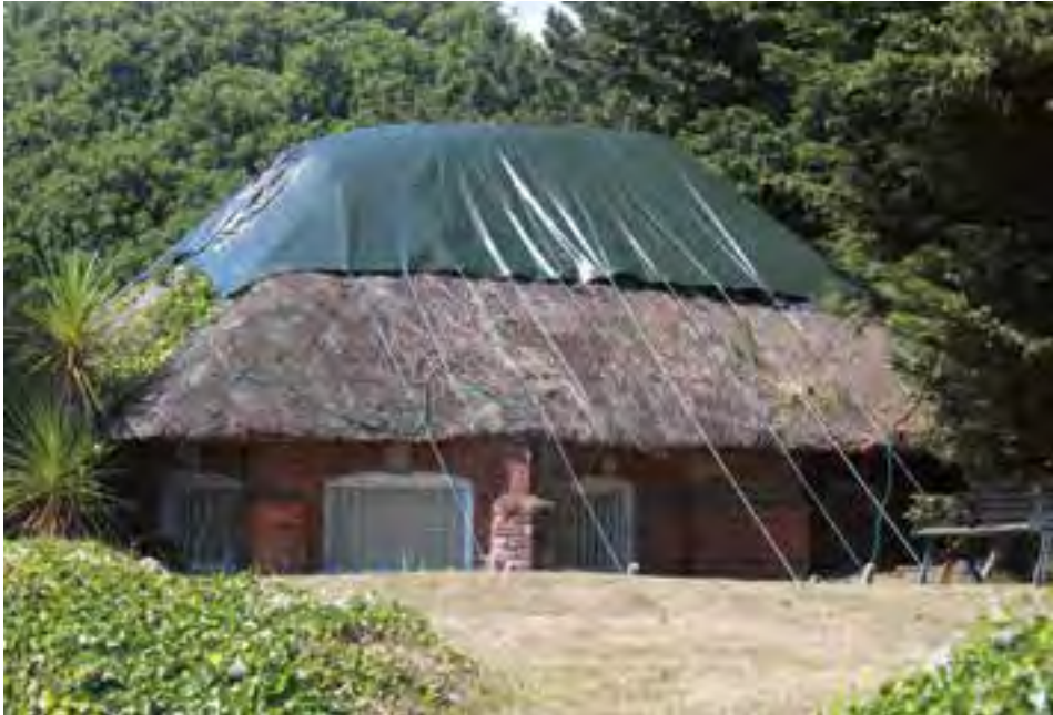
Figure 14. Former gun store for ECDB at Lowestoft.
