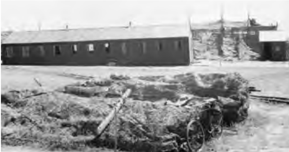
Figure 20. Kessingland Battery under construction in 1941. The camouflaging netting was standard by this date, as there was to be no sign from the air that construction was ongoing. (Imperial War Museum H11482)
